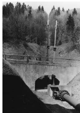
Penstock by control centre 2 View of the Born hillside
