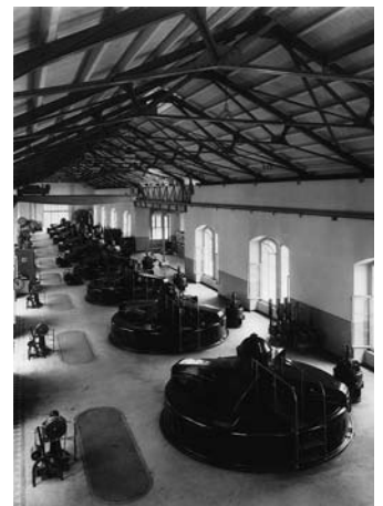
Generator room with new Brown Boveri generators
