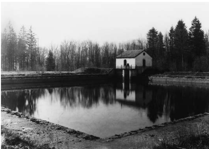
Reservoir on the Born for the high-head facility
