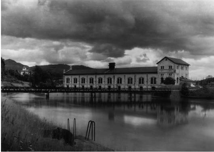
Powerhouse, viewed from upstream In the foreground: water catchment for the high-head facility
